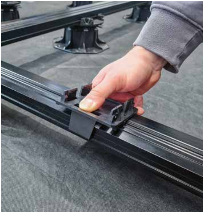
click the KL cross connector on to the aligned counter battens
