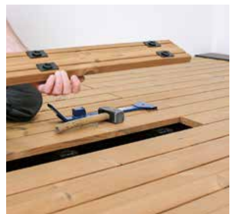
... and reinstall decking boards.
